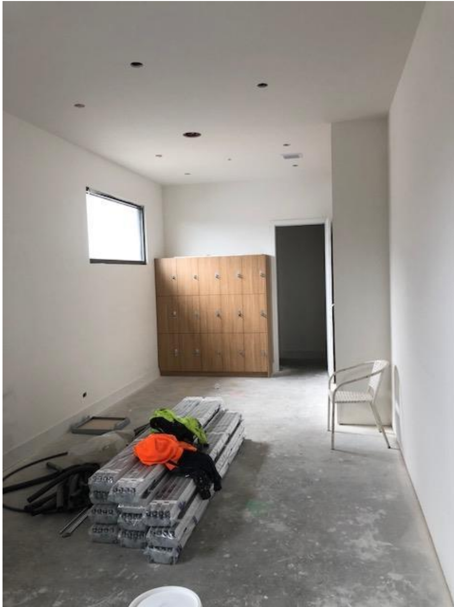
Figure 5 Ladies Locker Room
