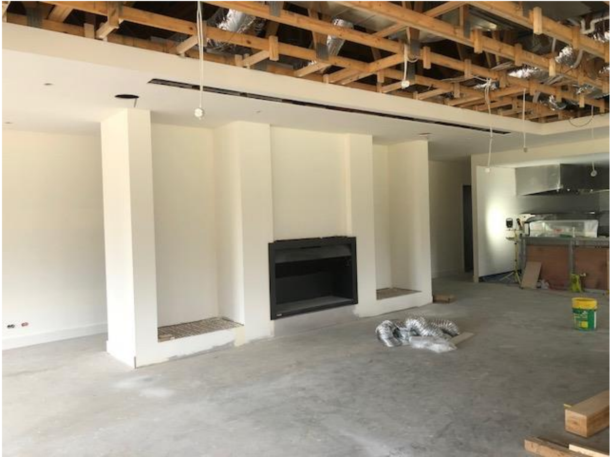
Figure 3 Members Bar Open Fireplace
